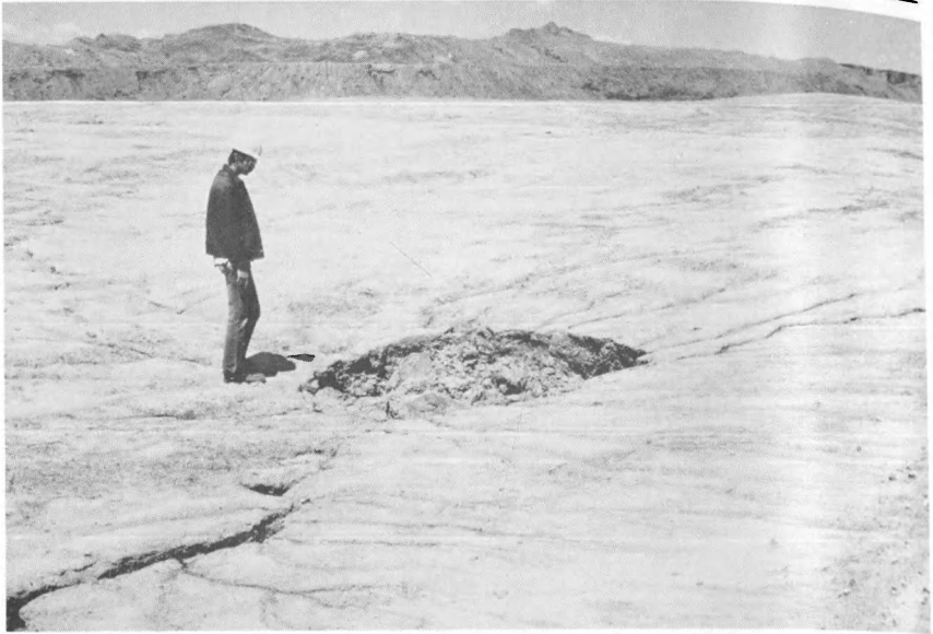
Figure 2. Collapse feature in spoils showing all surface drainage flowing toward the depression.
