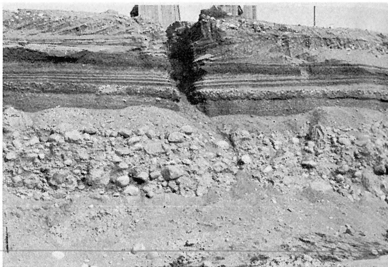
FIGURE 5—Armored mud ball layer in pit excavated for the Minute Man missile system.
